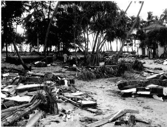
Figure 3: Buildings that were completely destroyed by the Tsunami (Photograph taken immediately after the tsunami) (photo: offered by the guesthouse owner)
