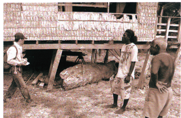
Figure 10: Photo of House 3 after the tsunami showing its leaning posts and the dead trunk of a Buni tree deposited beneath the floor (photographed by Sakamoto, on June 19, 2007).
