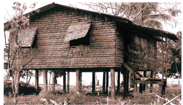
Figure 7: House 10: a typical house with raised floors with walls made of Sago palm fronds (photographed by Sakamoto, on June 19, 2007).
