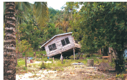
Photograph 1: Raised-floor dwelling of damage category 'impossible to reside'
